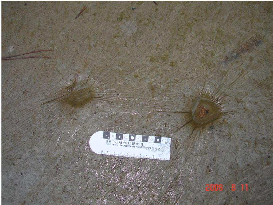
Fig. 8. A similar example of radial fractures around some unknown animal footprints preserved in wet concrete.
